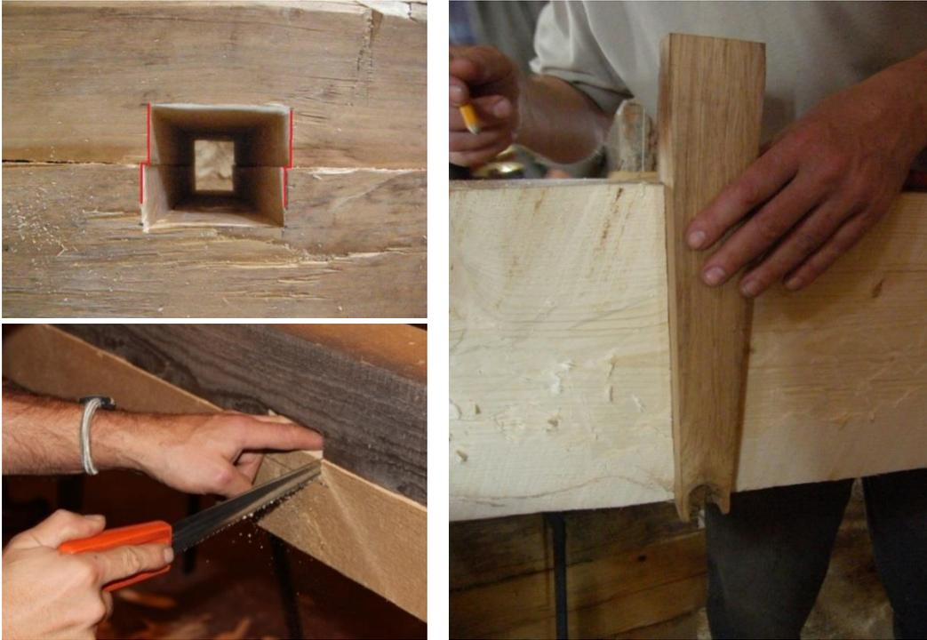
*Fig. 34 a) Cutting grooves for keys with offset allowing shoring of faces when tightening keys (highlighted in colour, top left), b) check of the key fitting in groove (right), c) formation of groove for key on the assembled joint (bottom left)*
