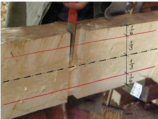
*Fig. 31 Undercutting two-thirds of the inner central part of the joint, contact surfaces remain only along the edges of the joint*
