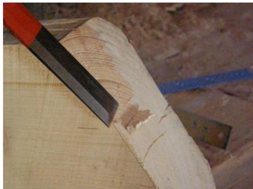
*Fig. 32 Cutting off the excess length of the scarf joint*
