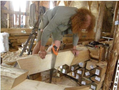
*Fig. 29 Preparation of a groove for a key using a hand saw*
