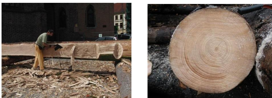
Fig. 42 Fine hewing (left), compression wood of spruce (right)
