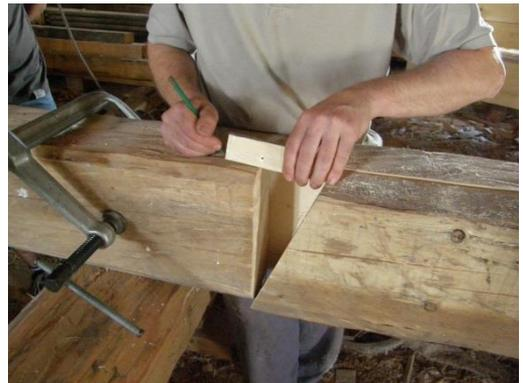
*Fig. 30 Marking the oblique face according to already prepared counterpart*
