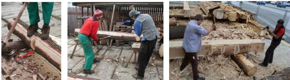
Fig. 41 Notching (left, centre) [16], rough hewing (right)
