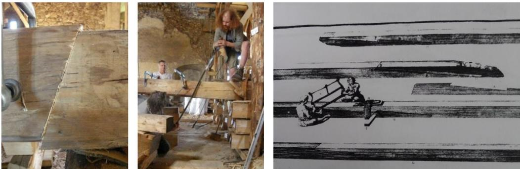
Fig. 33 a) Putting the joint faces together, b) cutting through by a handsaw c) cutting through the joint faces [19]
