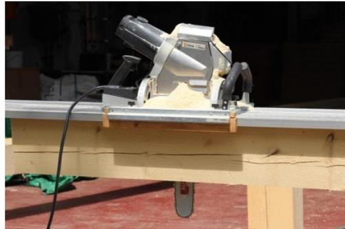
Fig. 22 Cutting a longitudinal scarf joint by a carpentry chainsaw
