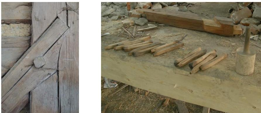
*Fig. 37 Wooden nail in the joint (left), wooden nails removed from the joint (right)*
